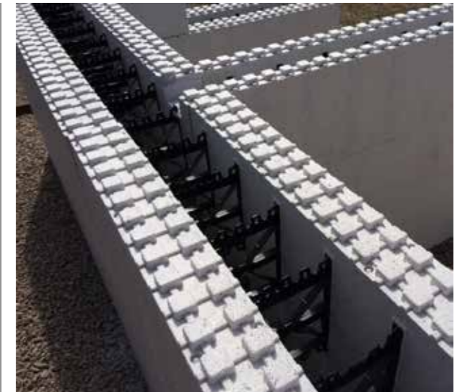
Horizontal armering i Thermomur 350.
